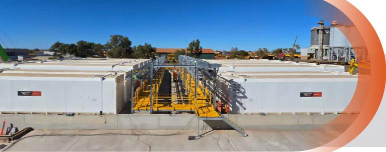
Our capabilities also encompass the supply and installation of structural steel pipe racks, walkways, canopies and gantries. Additionally, we provide supply and installation of self-bunded tanks with all interconnecting pipework. Our team is equipped to complete pipework and welding to various specifications, including AS4041, utilising in-house qualified welders supported by dedicated QA/QC processes to ensure high-quality, reliable deliverables.
