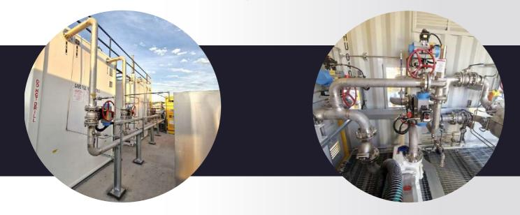
Project works also involve installation of 16 Ebsray HD400 gear pumps and 10 316SS fabricated filter vessels. Our team leverages proven expertise in large-scale concrete work, piping, structural steel installation, and advanced fluid handling systems to deliver these acomplex and demanding facilities efficiently and to the highest standards.
