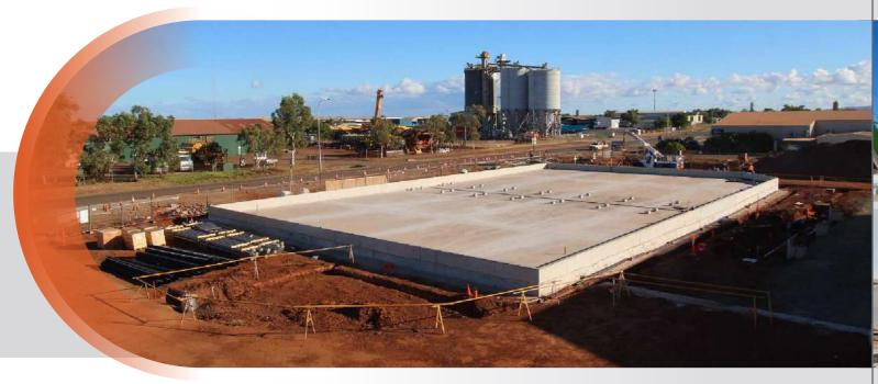
The current Karratha project undertaken by Ngpetro includes all of the aforementioned scopes, with a focus on extensive fluid storage and fluid handling systems. This project features the construction of 2.4 million litres of lubricant storage capacity, connected via approximately 1.2 km of 316SS pipework, primarily 4" and 6" in size.
